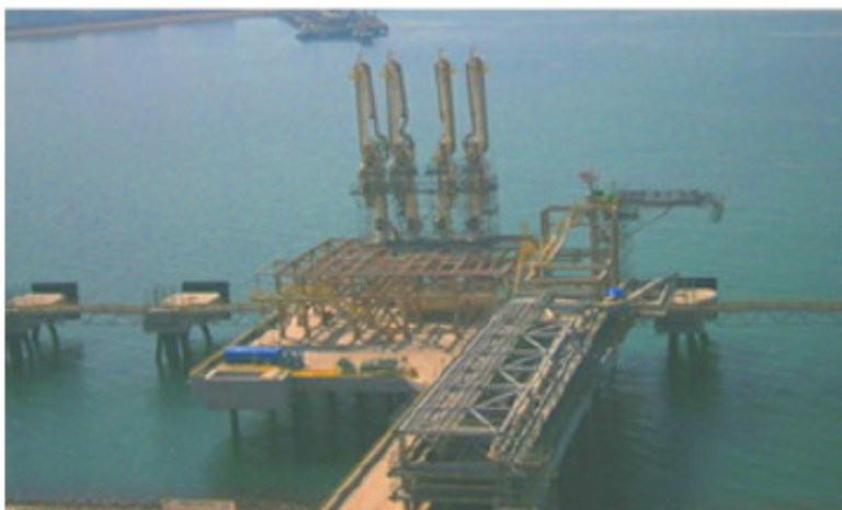
Approach bridge and jetty head
