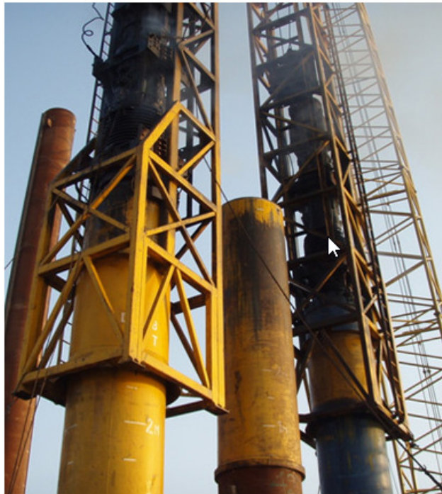
Driving of steel pipe sheet pile using suspension hammers
