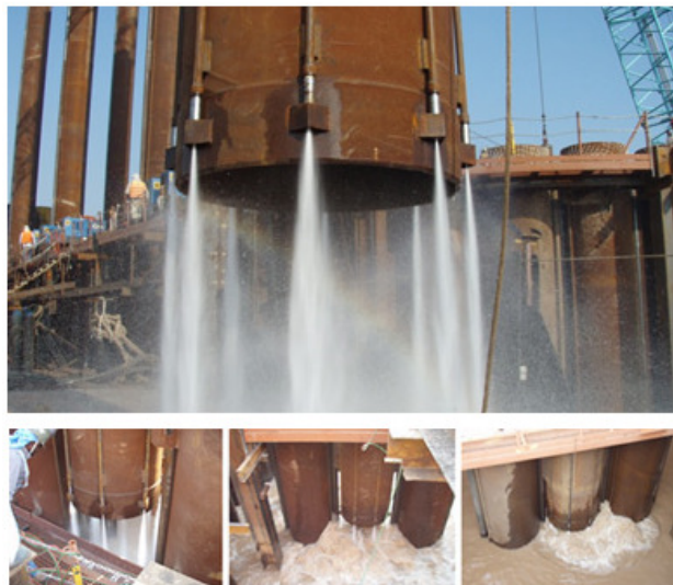
Installation of steel pipe sheet pile with hi-pressure water Jet system
