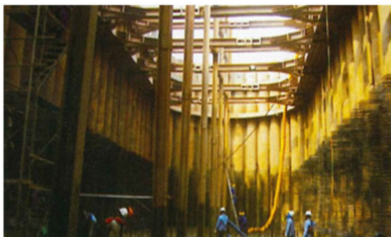
Internal view of cofferdam
