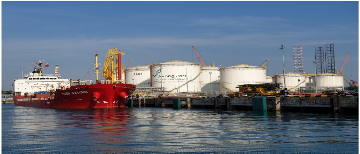
Upgraded Berth J18 and J19 receiving first vessel on 17 th March 2019
